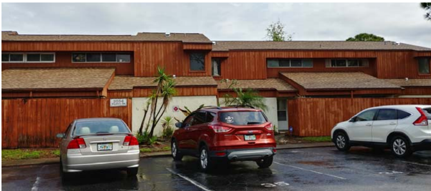
New Roof Is Looking Good !!!
